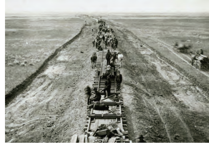
Track is laid across virgin prairie in Dakota Territory during the record-breaking year of 1887.
