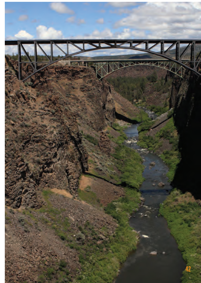
The Crooked River Bridge in Oregon was the highest arch bridge in the U.S. when it was built in 1911, spanning a canyon 320 feet deep and 350 feet wide.
