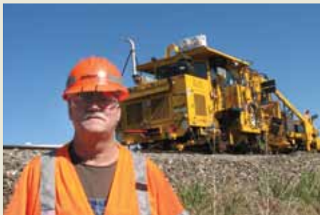
Mike McMahan was the first to operate the new tamper.
